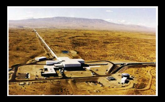
Located in Hanford, Washington, this is one of several gravitational wave (colloquially, gravity wave) detectors around the world. It has two perpendicular arms, each 4 km long. Gravity waves that pass the detector cause unequal changes in the lengths of the arms. These changes are detected by lasers inside each arm.
