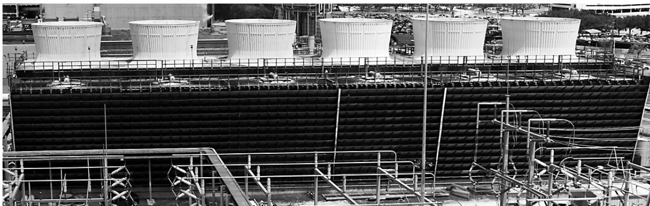
Figure 11.2 A mechanical-draft cooling tower. The fans are located within the cylindrical housings at the top. Air is drawn in through the louvers on the side.
