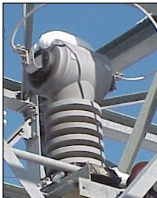
Current Transformer in Switchyard.
