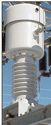
Current Transformer in Switchyard.
