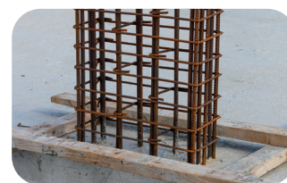
Fig. 4.12 Reinforcing concrete
