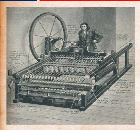
Machinery like the cotton spinning jenny was designed to be used by child workers with their small build and nimble fingers. Children were often employed in textiles factories because they were small enough to move between tightly packed machinery.
