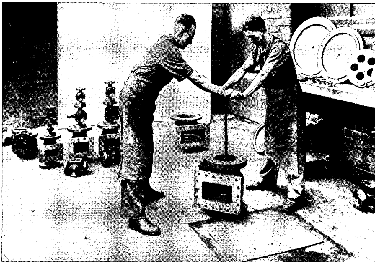
"Method of Lapping Seat in Valve Body"
