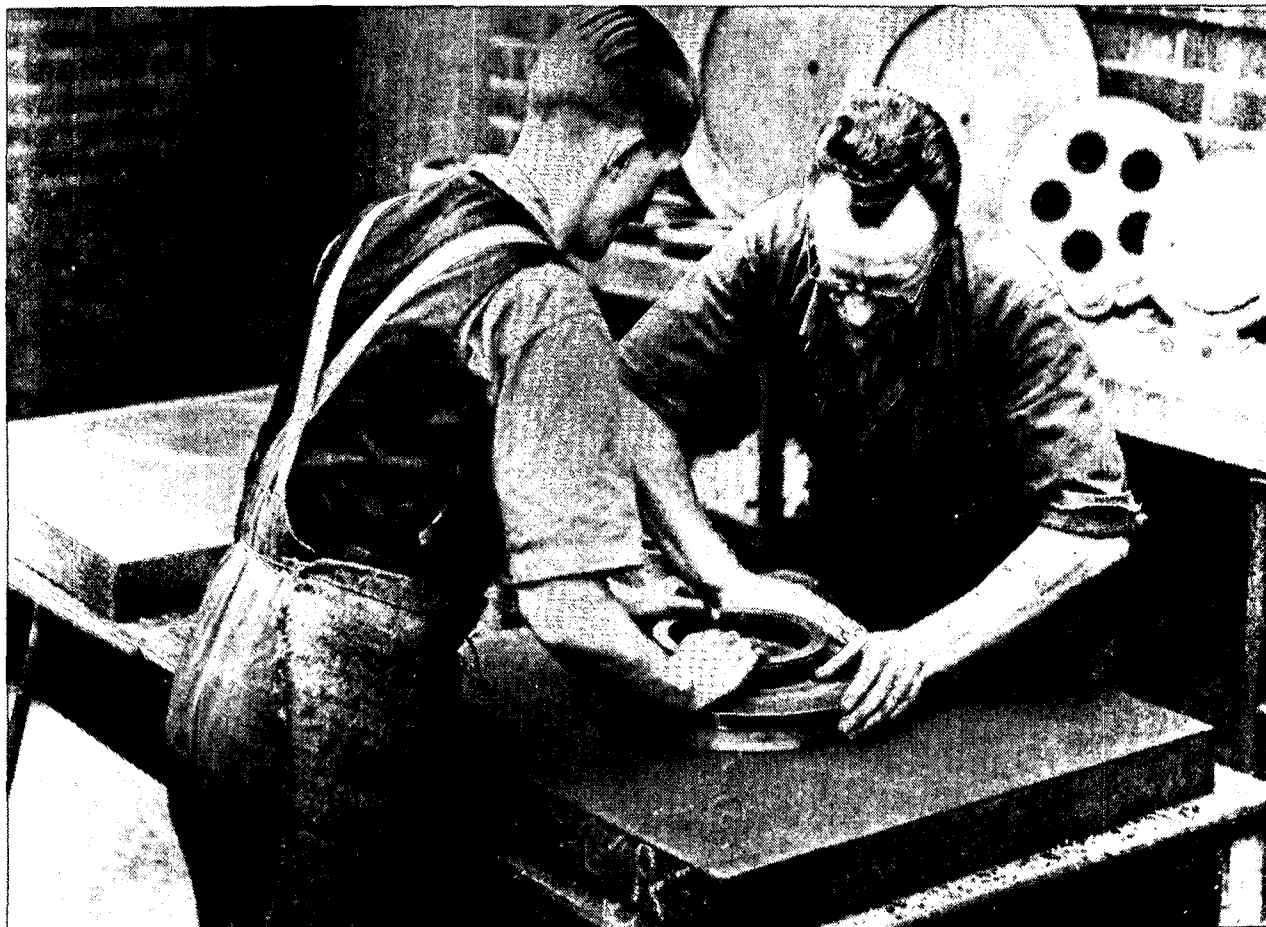
"Lapping a Large Valve Disc"
